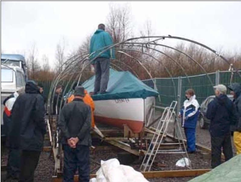
Erecting the poly tunnel hoops in the rain! Oh! for the Cowshed at Beale Park
